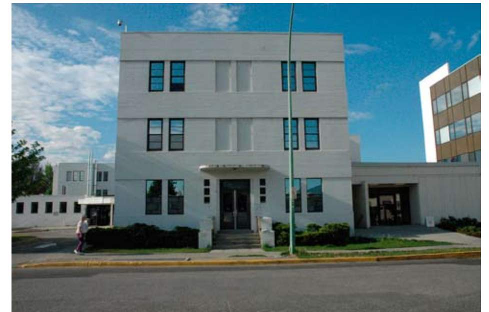
Pandosy Building East Face
