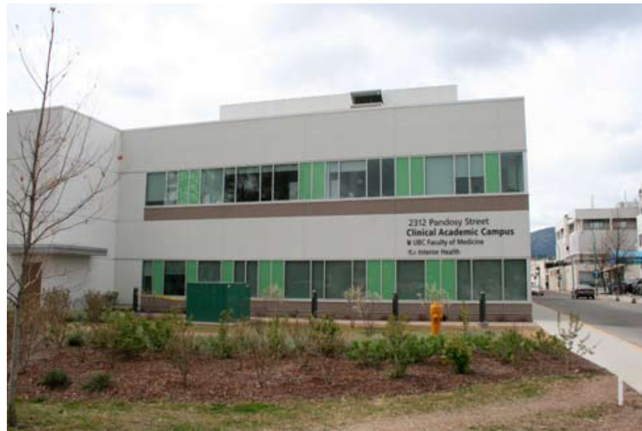
CAC East Facade
