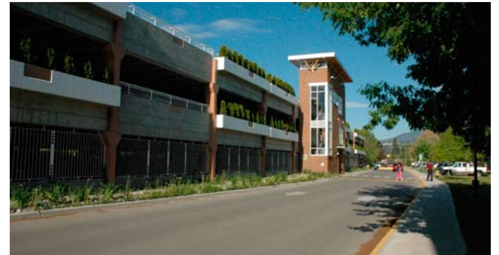
View of Existing Parking Structure
