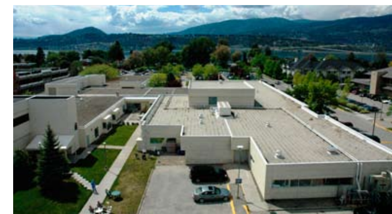
View West of Abbott Building
