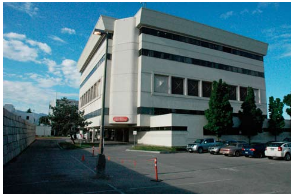
Royal Building North and West Face
