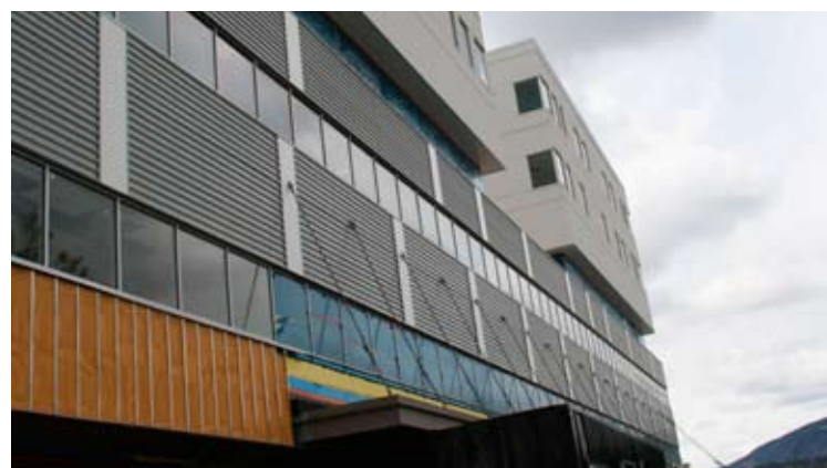
CEN Under Construction
